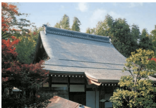
Figure 3. Koetsu-Ji Temple in Kyoto with titanium sheeting imitating burnt tile
